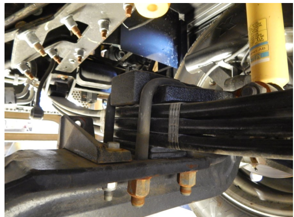
U-bolts will be reused
