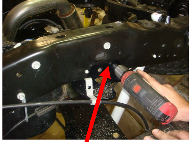
Drivers side upper air bag mount Two 1/2" hole needs drilled
