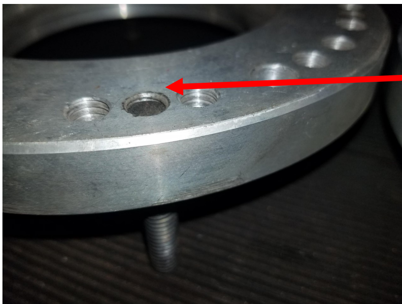
Correct stud length after installation
